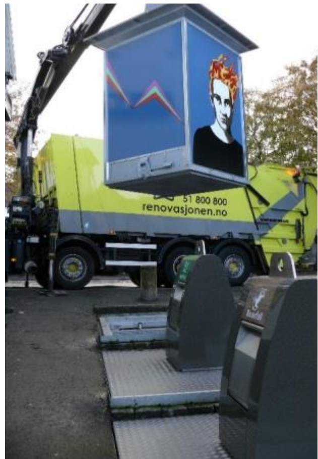
Emptying of underfloor container
