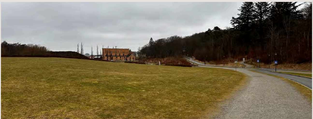
The culvert (both photos)
